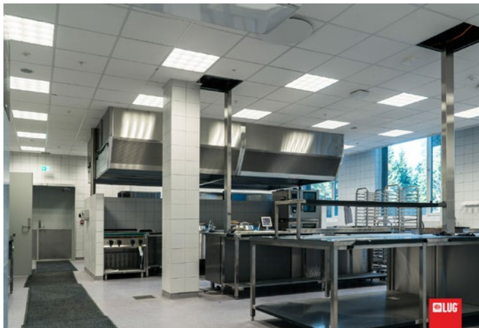
LHL Hospital, Oslo, Norway
